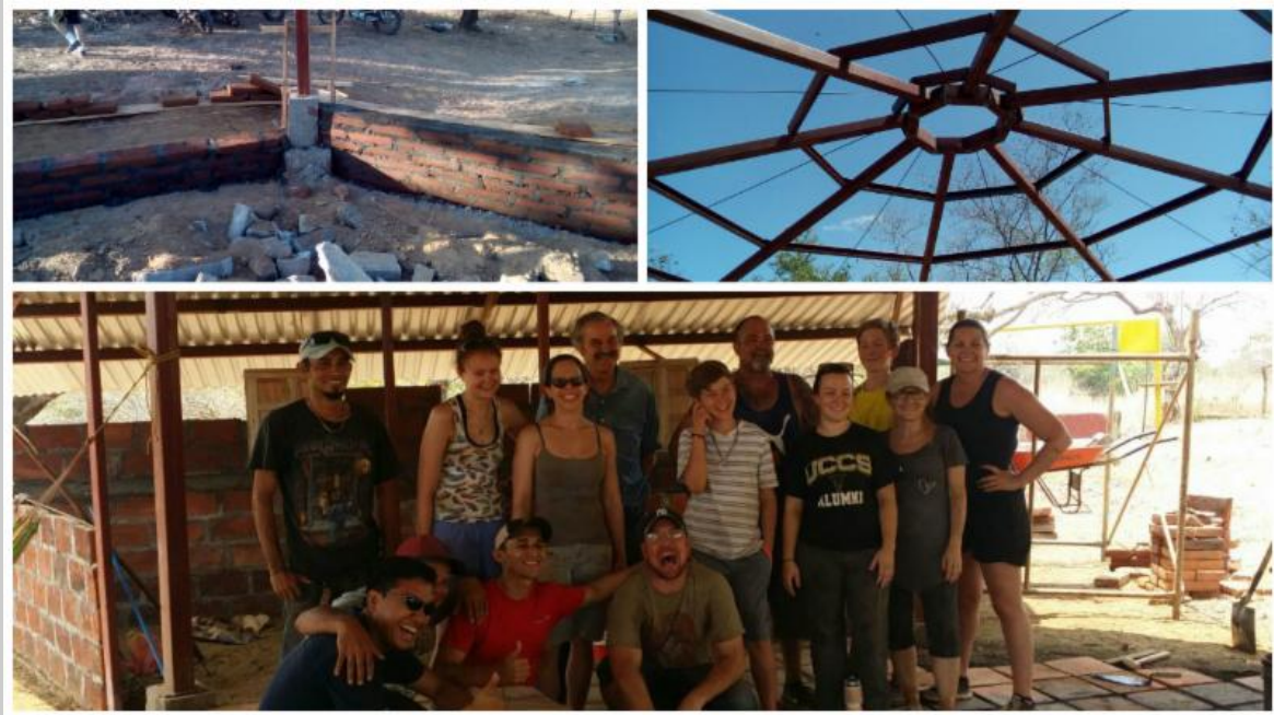
Our Colorado Partners working hard on the Learning Center.
